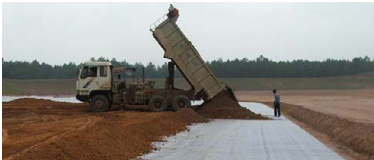
▲ Geotechnical materials used for consolidating road grounds in weak soil structure such as wetlands, dykes, irrigation systems and embankments
